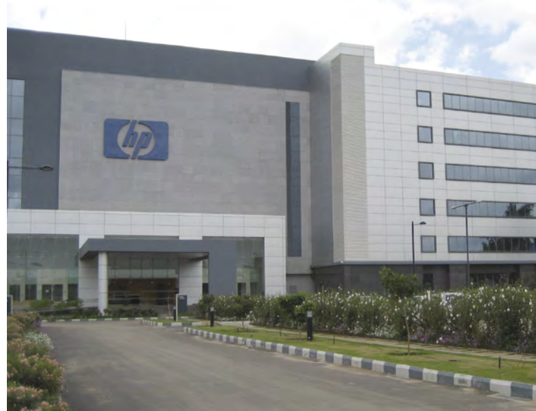
HP R&D Laboratory Data Center
